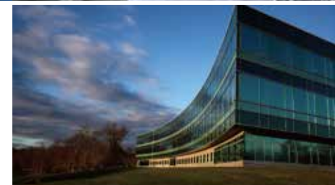
New Jersey R&D center
