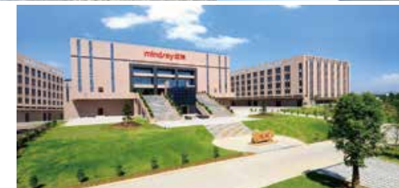
Manufacturing center in Shenzhen
